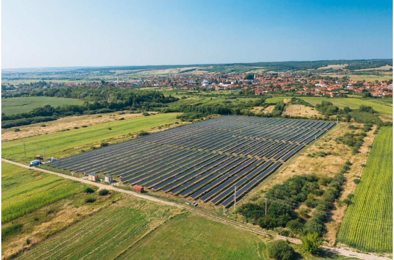
3,2 MWp solar PV power plant Făget 1 | Image source: Photon Energy Group
